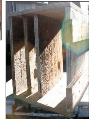
Placement of baffles inside the bat roost.
