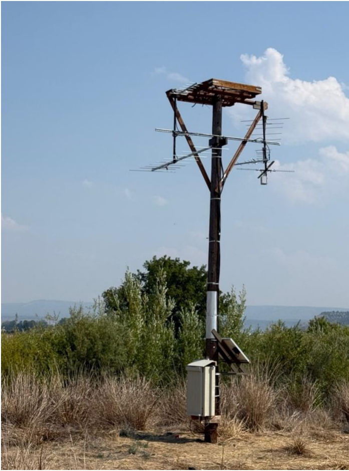
Osprey nest pole with 7 antennas and the SensorStation cabinet and solar panel.
